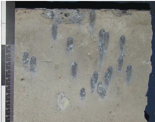
Fig. 4. Damage to the concrete block caused by ricochet of 5.6 mm lead bullets
