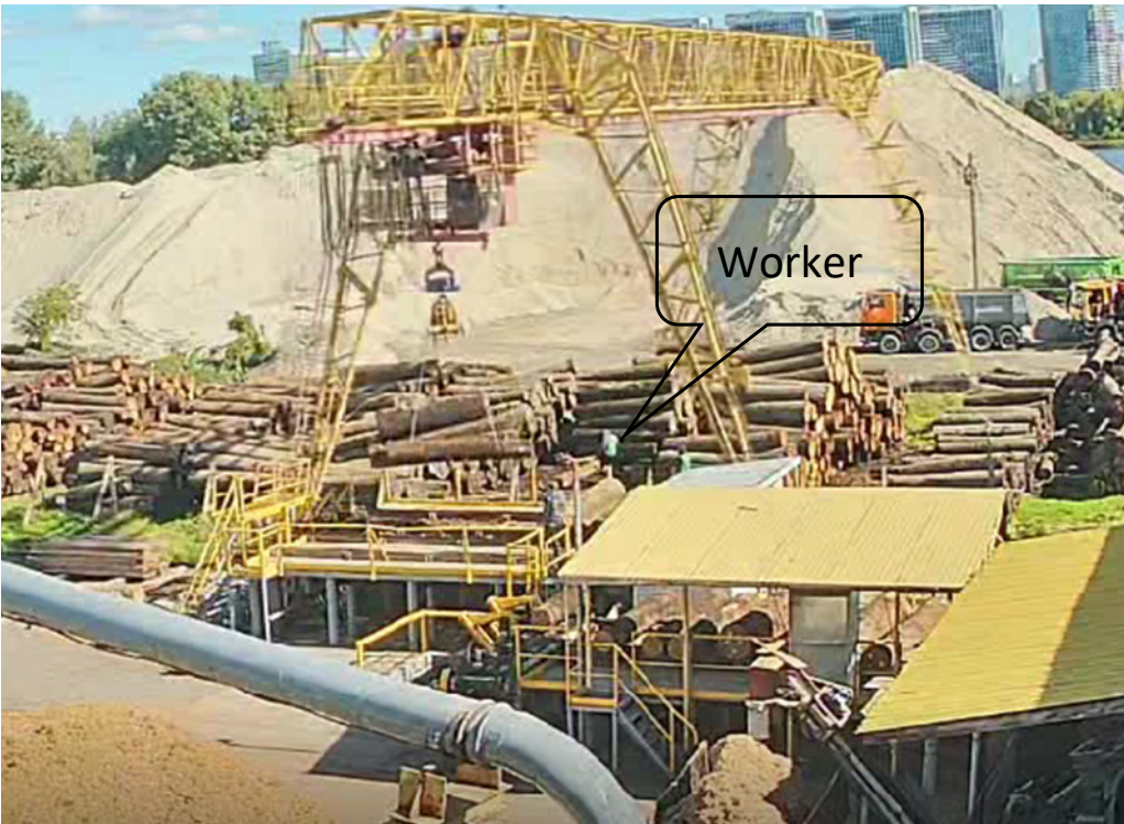
Fig. 7. Circumstances of the accident at a timber processing plant involving safety violations
