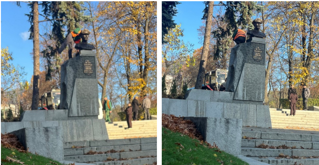
Fig. 2. Performing work on the monument in violation of health and work safety requirements
